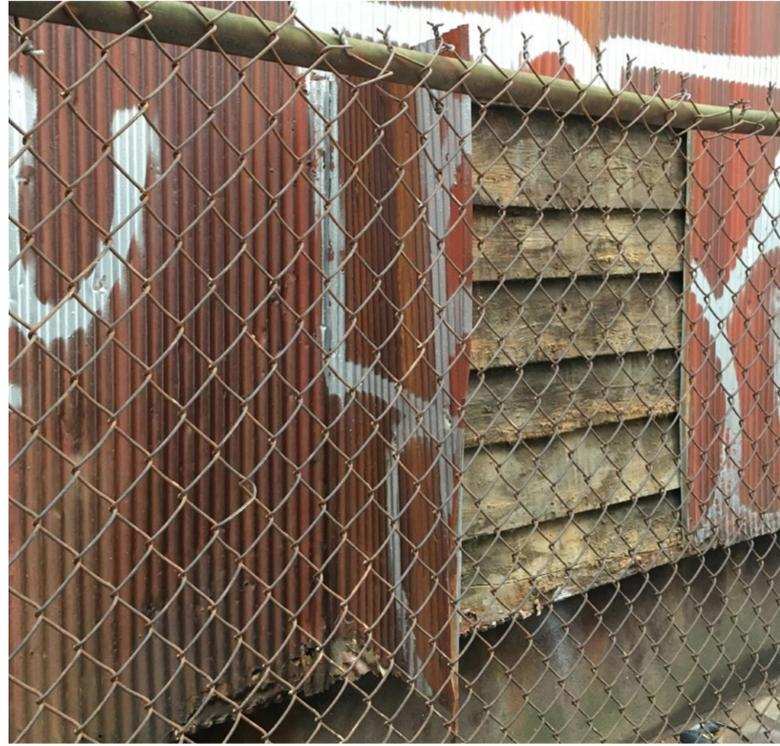
view of clapboard siding under metal panel
